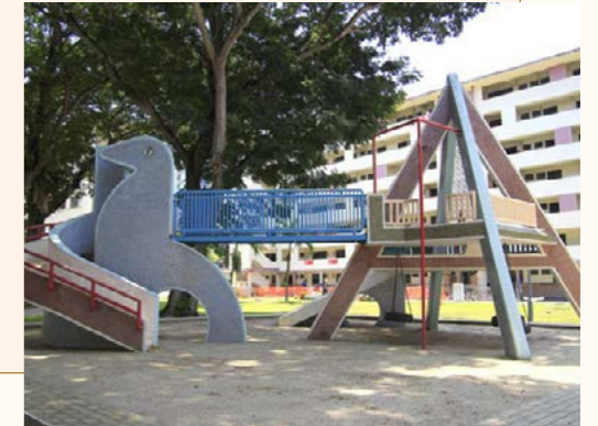
Residential blocks to be conserved and Dove Playground to be kept as identity markers at Dakota Crescent. SOURCE: URA
