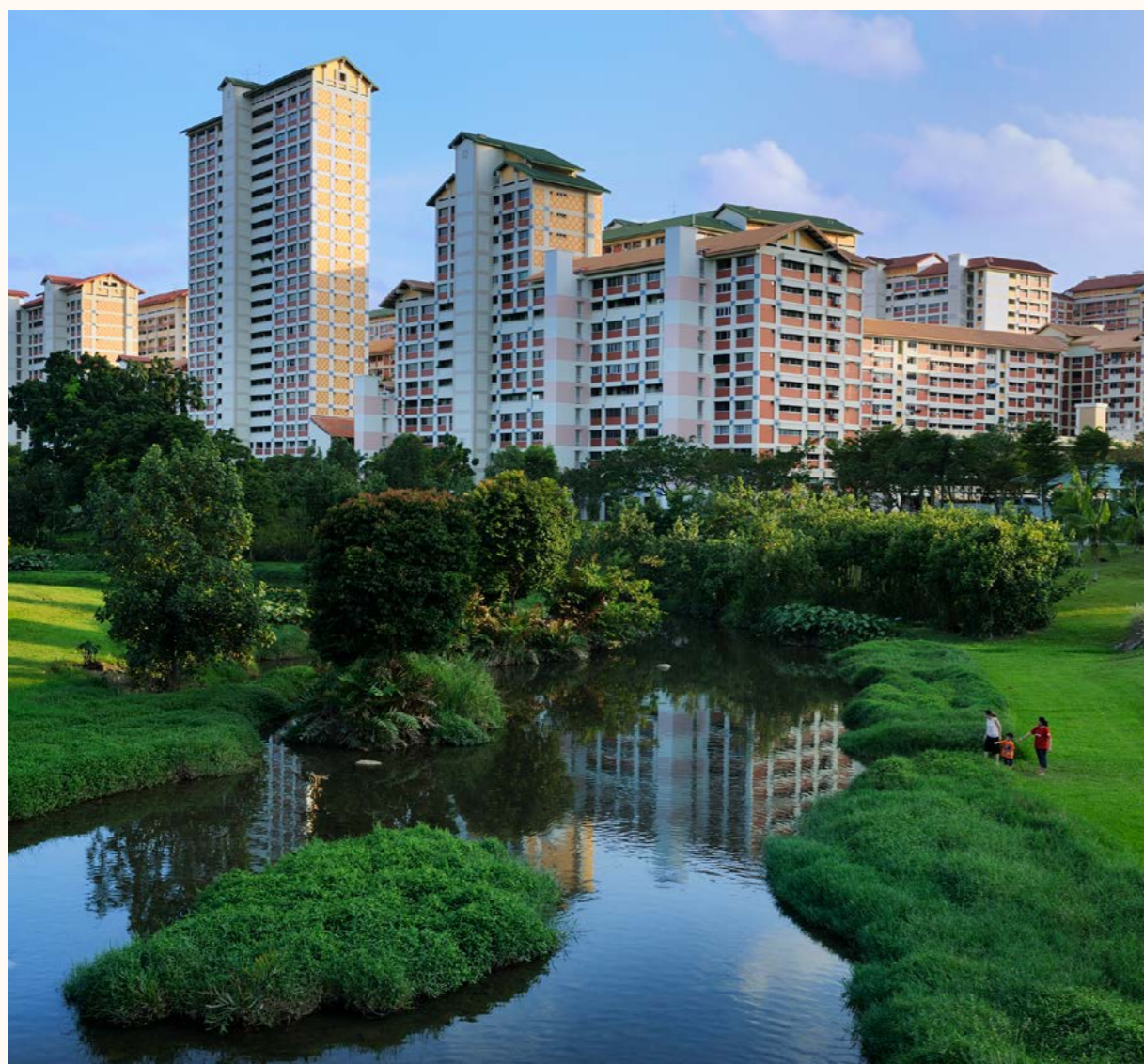
Housing overlooking Bishan-Ang Mo Kio Park. SOURCE: NPARKS
